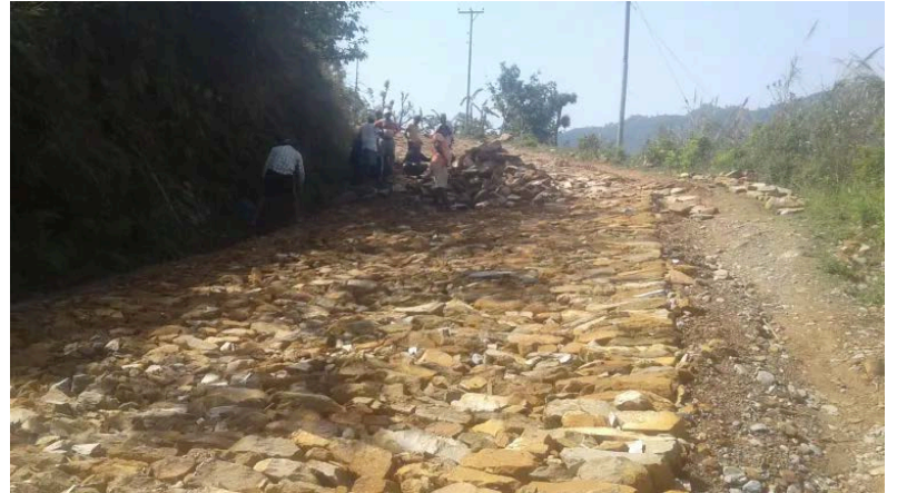
Paving of the road by the villagers
